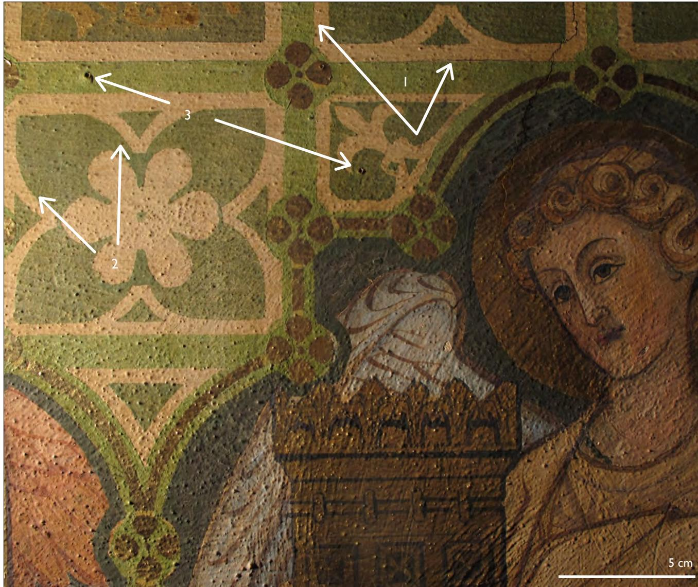
Several methods of setting out used on the chancel dado: Green grid painted first, using stencils and pencil lines (1). Squares filled in with stencils, as shown by lips of paint where stencil was lifted off (2). Tack marks through tile paint (3) suggests figurative quatrefoils were painted after tiles. Indicates quatrefoils transferred from full scale drawings.
